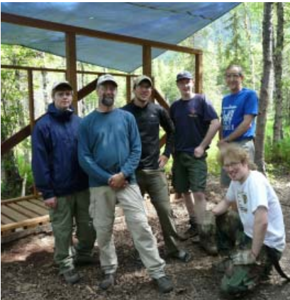
Thank you to Scout Simon Kiehl and his troop for raising funds, designing, and building a wood storage shed (June 2011). Job well done!
